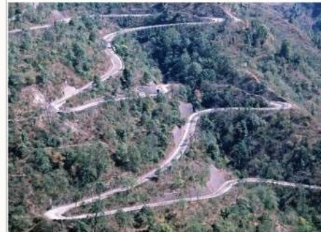
b) Extensive use of gabion retaining walls to support road fill and revetments to protect cut slopes
