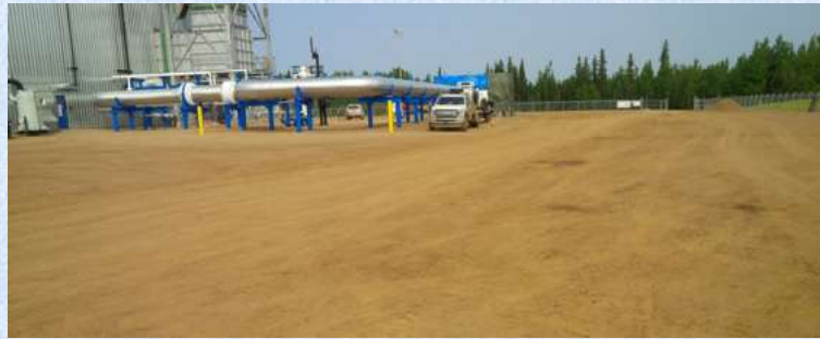
After one and a half year in operation
