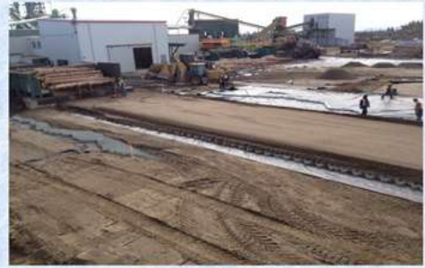
Portion of completed surface
