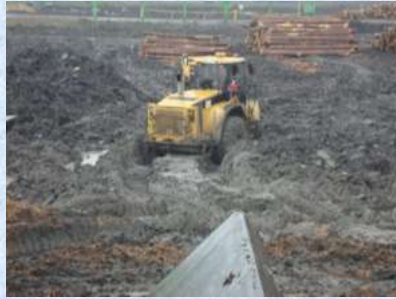
CAT 988H before construction
