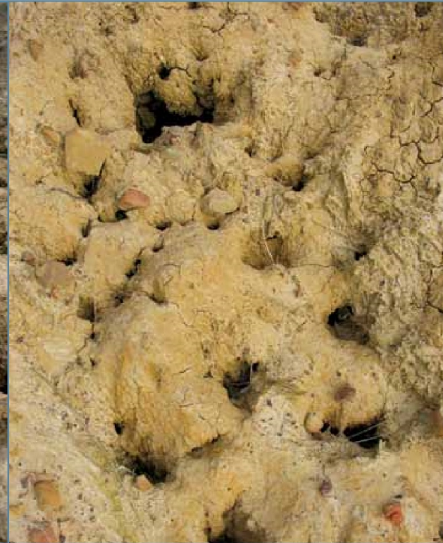
ilting from topsoil removal, surface water has dissolved through the soil surface. Soils derived from Triassic
