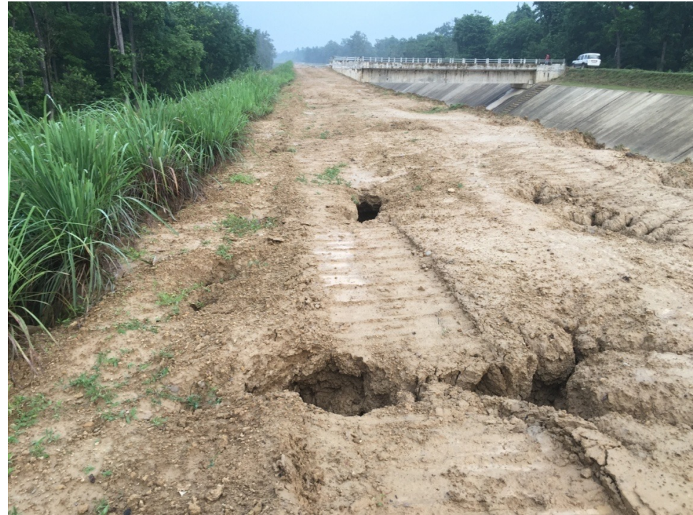
Jugholes found in the Embankment Top and Canal Berm
