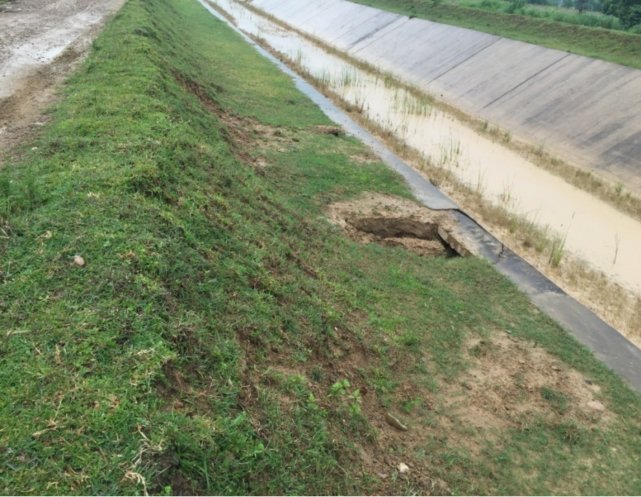
Jugholes found in the Embankment Top and Canal Berm
