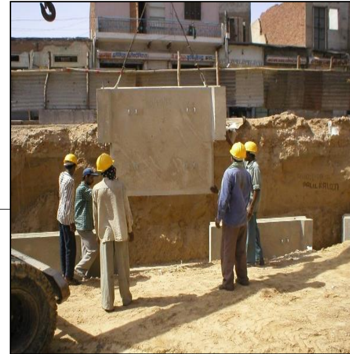
PLACEMENT OF FIRST ROW PANELS
