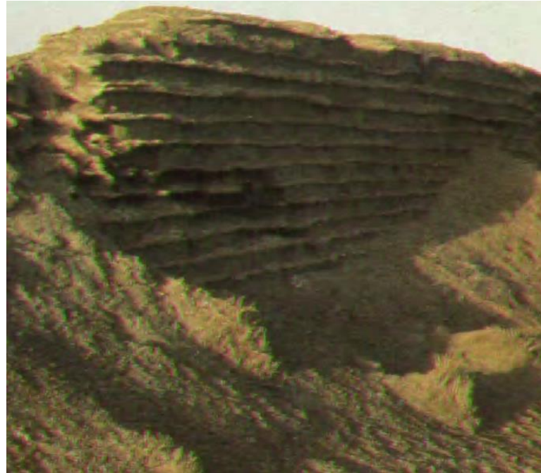
Ziggurat- Reinforced Soil Structure using Natural Straw
