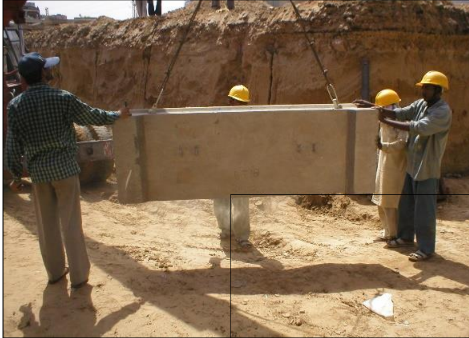
PLACEMENT OF FIRST ROW PANELS
